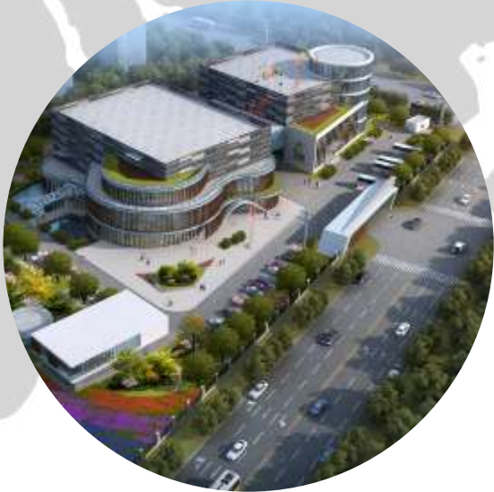
New China Campus (Coming Soon)
